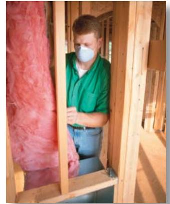
**Safety First** A worker must always use the proper safety equipment when installing insulation. *Why is this worker wearing a breathing mask?*
